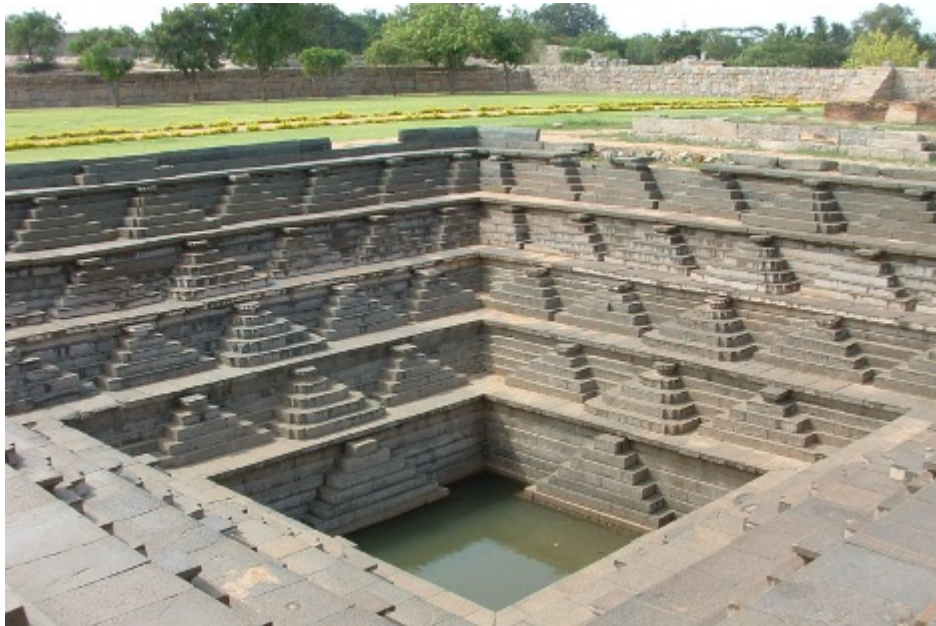
Fig. 1: Vijayanagara. Chalukya-period stepped tank of chloritic schist in the Royal Centre (Richard M. Eaton)
