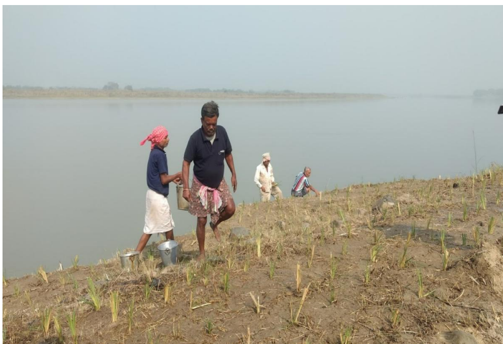
Example of MGNREGA work: Vettiver planting to prevent soil erosion, Nadia, West Bengal, December 2016 | Sudha Narayanan
